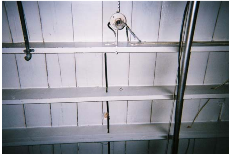
Figure 1. Waiting on pain - View when looking at ceiling
